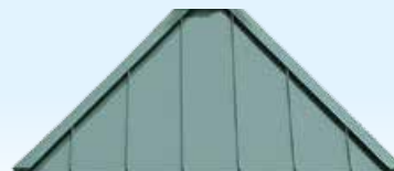
Standing Seam Metal Roof
